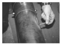
Line up holes in duct and secure with bolt and nut provided.
