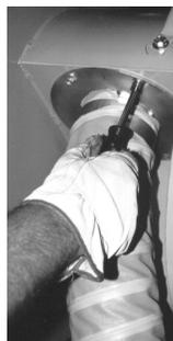
Make sure gasket is in place between tube and reel flange
