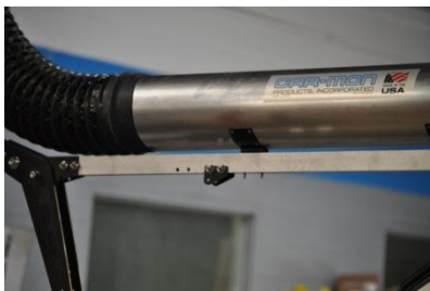
Illustration C: Duct connection aluminum support structure; secure with ¼-20 whiz-lock nuts
